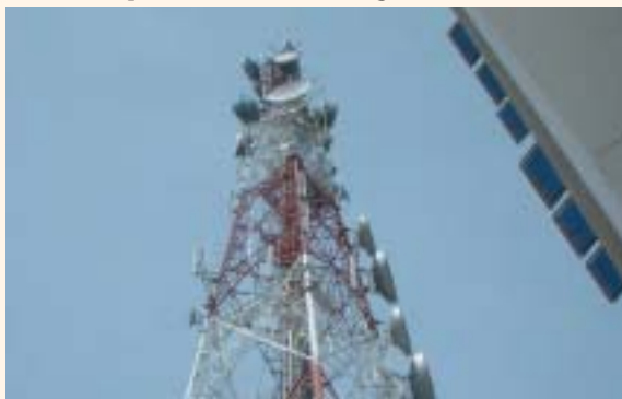
The transmission tower in Ayutthaya
