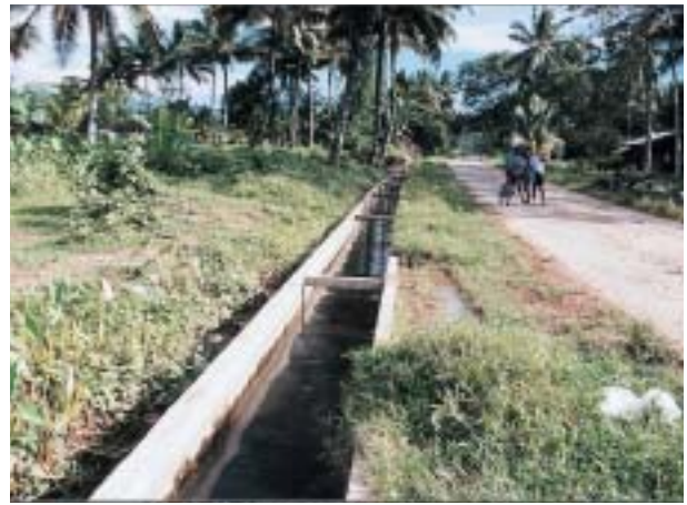
A Network of Branch Irrigation Canals and a Market Access Road
