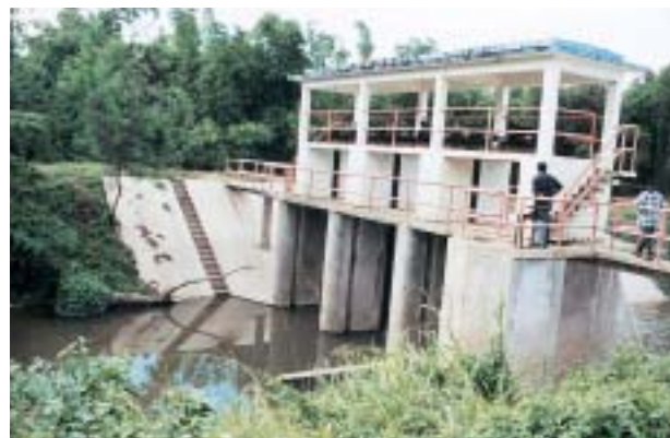
Water Intake Dam Constructed by the Project
