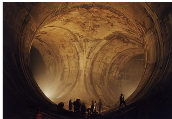
Diverging Point of Intake Tunnel
