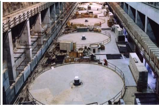
Underground Turbine Facilities
