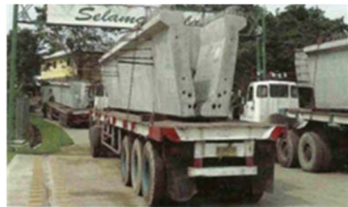
Figure 6.4-4 Precast PC-U Girder and Transport of PC-U Girder
