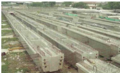
Figure 6.4-4 Precast PC-U Girder and Transport of PC-U Girder
