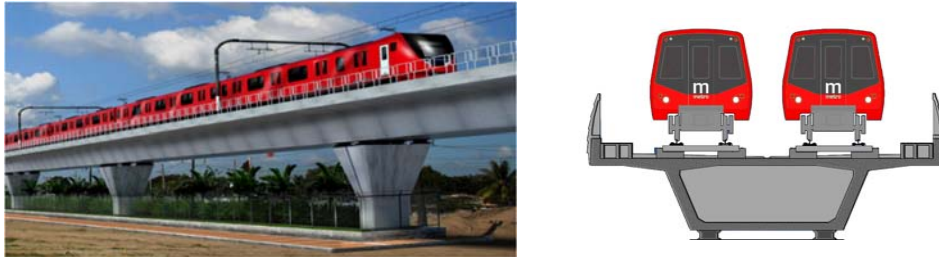
Figure 1.4.1 PC segmental box girder
