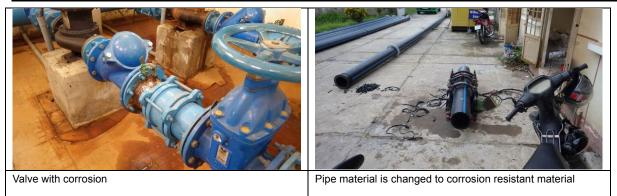
Figure 2.3.20 Damage to Water Supply Plant from Saline water intrusion Source: JICA survey team (2016)
