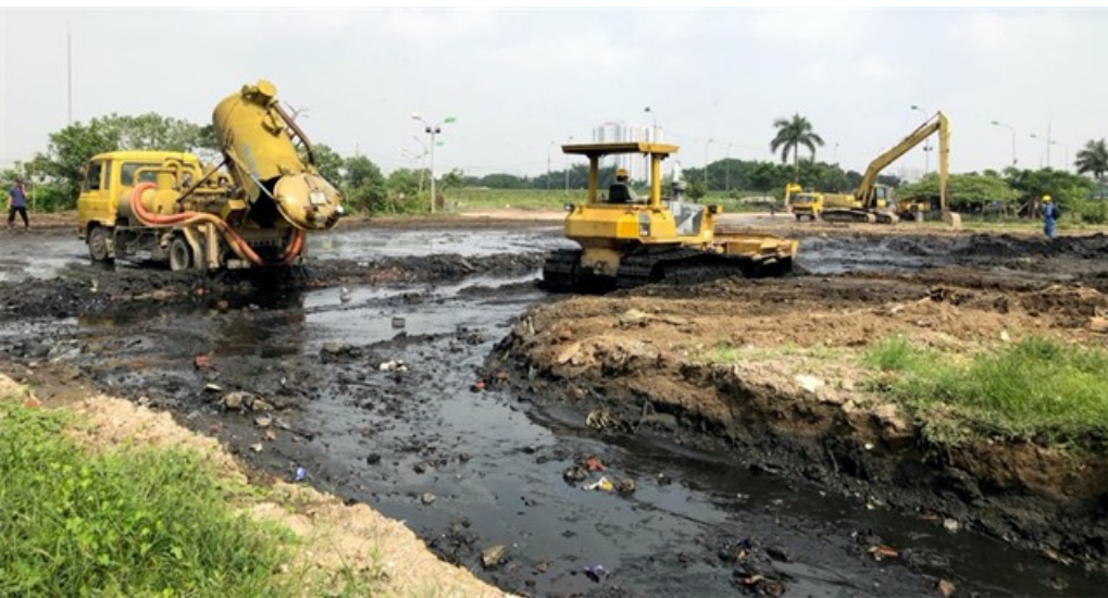
Yen So Backfilling Site of Hanoi Sewerage and Drainage Company (22 Aug. 2018)
