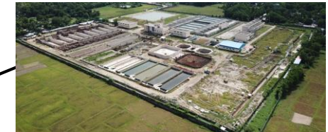
Karnaphuli water purification plant
