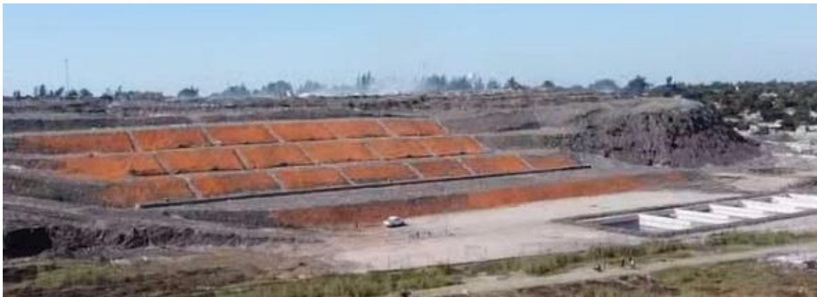
Completion of phase 1
