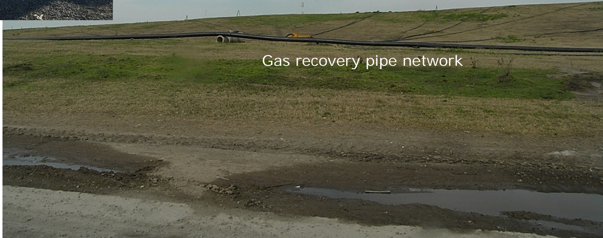
Methane gas recovery from anaerobic landfill (CDM project, Buenos Aires, Argentine)
