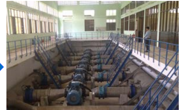
Replacement of pumps at water purification facility (Joint Credit Mechanism-supported project)
