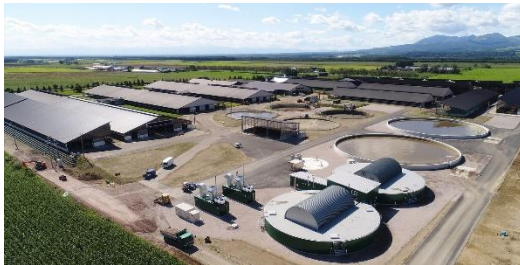
Biogas power generation facilities
