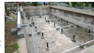
Installation of aerator
