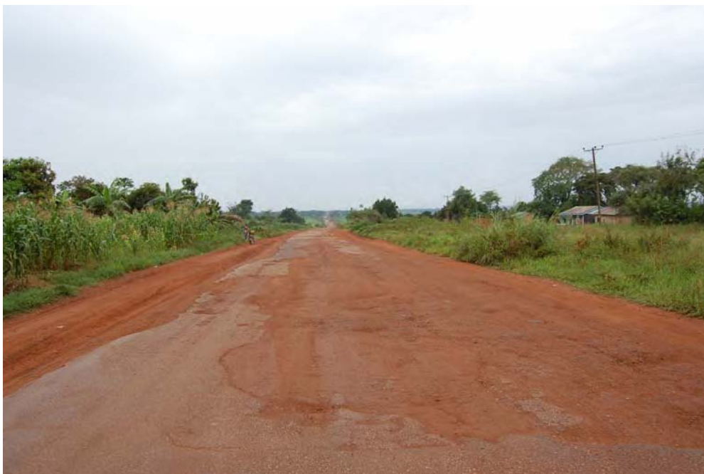
Note: Asphalt pavement was removed. Source: The Study Team
