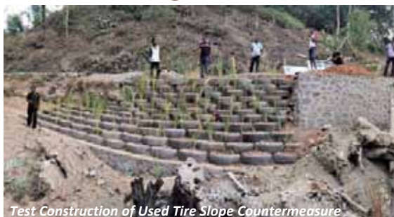
Test Construction of Used Tire Slope Countermeasure
