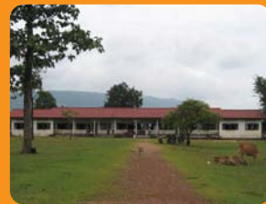
A schoolhouse constructed using grant aid cooperation (Madagascar)
