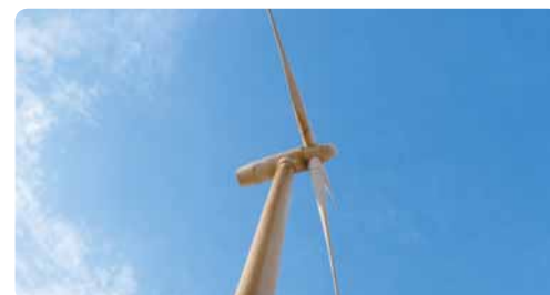
Wind generator constructed via ODA loan (Egypt)
