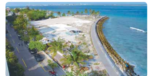
A coastal revetment on Malé Island constructed to reduce tsunami damage (Maldives)
