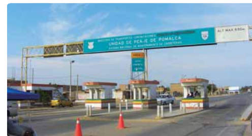
Contribution to rural economic development by building roads stretching from the interior to coastal areas (Peru)
