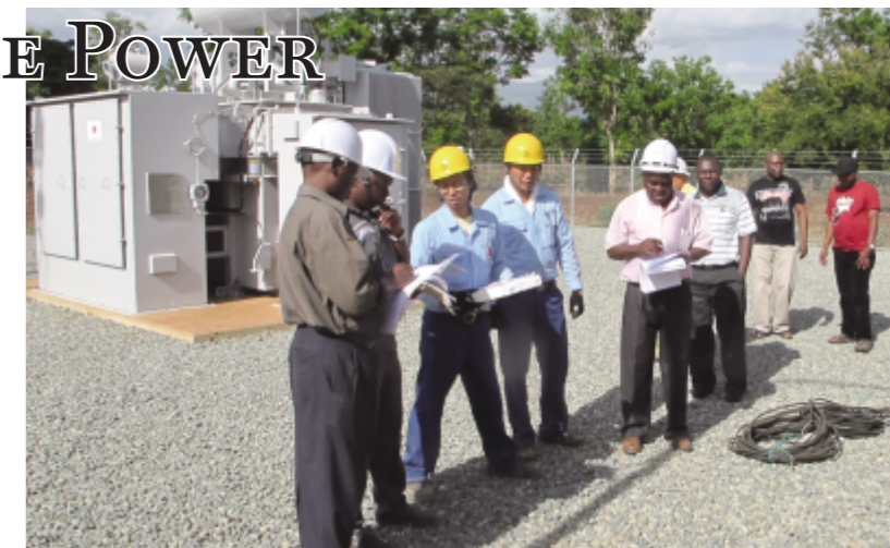
Japanese and Tanzanian experts make a final inspection before the inauguration of a new electricity substation in Kilimanjaro.
