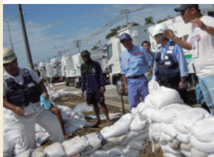
Pumping operations guided by Japanese engineers and using drainage pump cars
