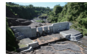
A sediment dam constructed on Mount Merapi
