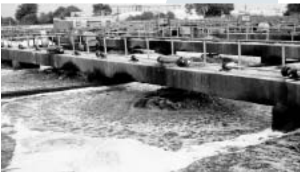
Sewage treatment operations at the Yamuha River basin community (India)
