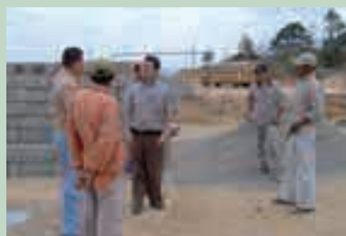
Construction site of a primary school, which is assisted by the project with the participation of the community
