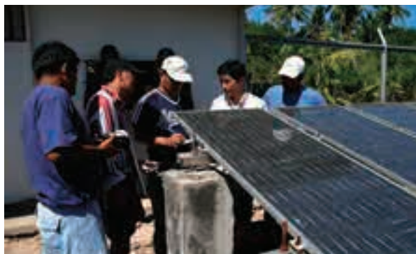
On-site training for maintenance and management of photovoltaic devices (The Project for Sustainability Improvement of Renewable Energy Development in Village Electrification, the Philippines)
