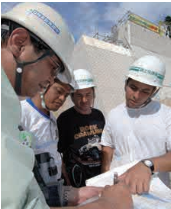
Training participants touring a mudslide-control dam under construction in Kobe City (Volcanology and Comprehensive Sediment-related Prevention Measures, JICA Tokyo) (Photo by Kenshiro Imamura)
