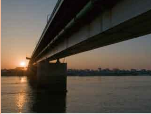
Chroy Changwar Bridge (Japan Bridge)
