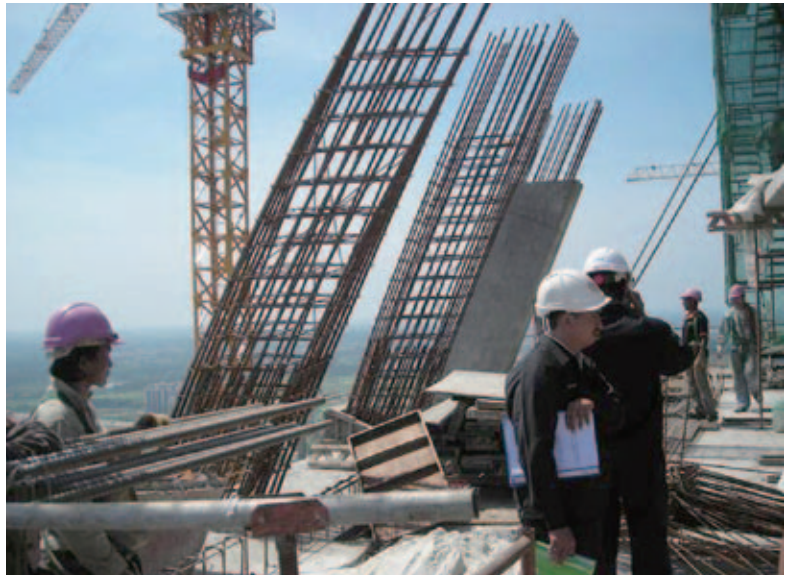
Hands-on training on safety supervision at a construction site (Project for Improving Occupational Safety and Health Administration of Department of Occupational Safety and Health of Malaysia)
