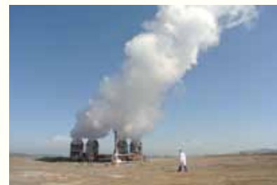
Geothermal steam production testing in Menengai, Kenya
