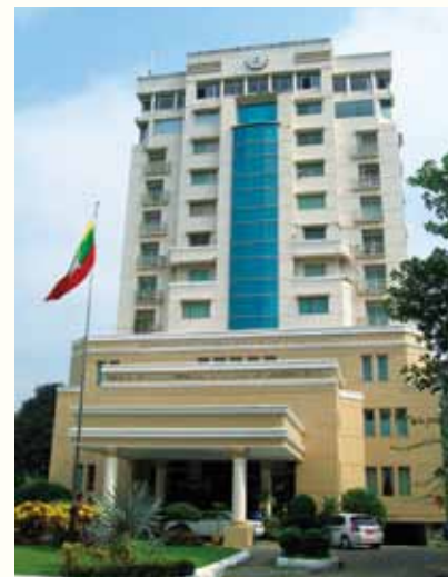
The Myanmar-Japan Center for Human Resources Development is located in the UMFCCI building.
