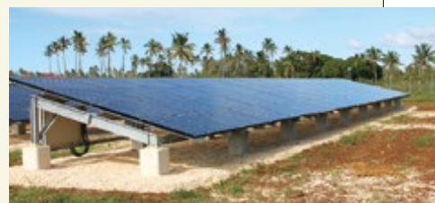
A solar power generation facility in Tonga
