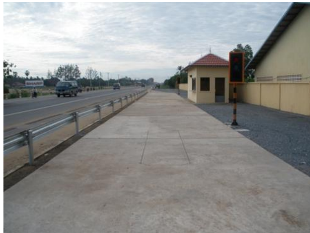
Figure 1.7 Truck scale after completion
