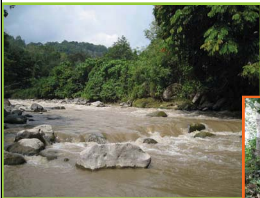
View of the power house point from the 2km downstream
