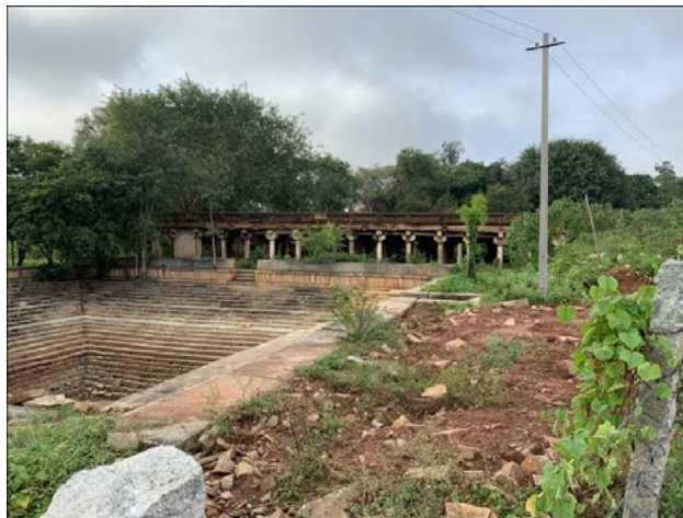
Figure 11: Most vibration sensitive structure in the project area – Chikkajala Old Fort and Temple @26+574km, 26.35m away, phase 2b
