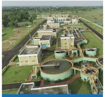
Aerial View of the Sewage Treatment Plant SD-II under the Odisha integrated sanitation improvement project. JICA's assistance is to support construction of three Sewerage Treatment Plants (STPs), with a total capacity of 100 Million Litre per Day (MLD).
