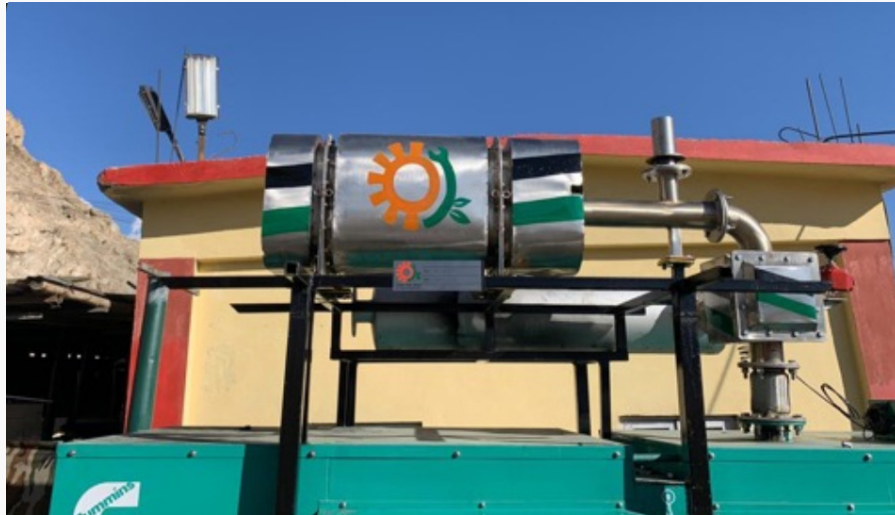
Chakr Innovation - Emission Control Device for Diesel Generators under the Neev Fund
