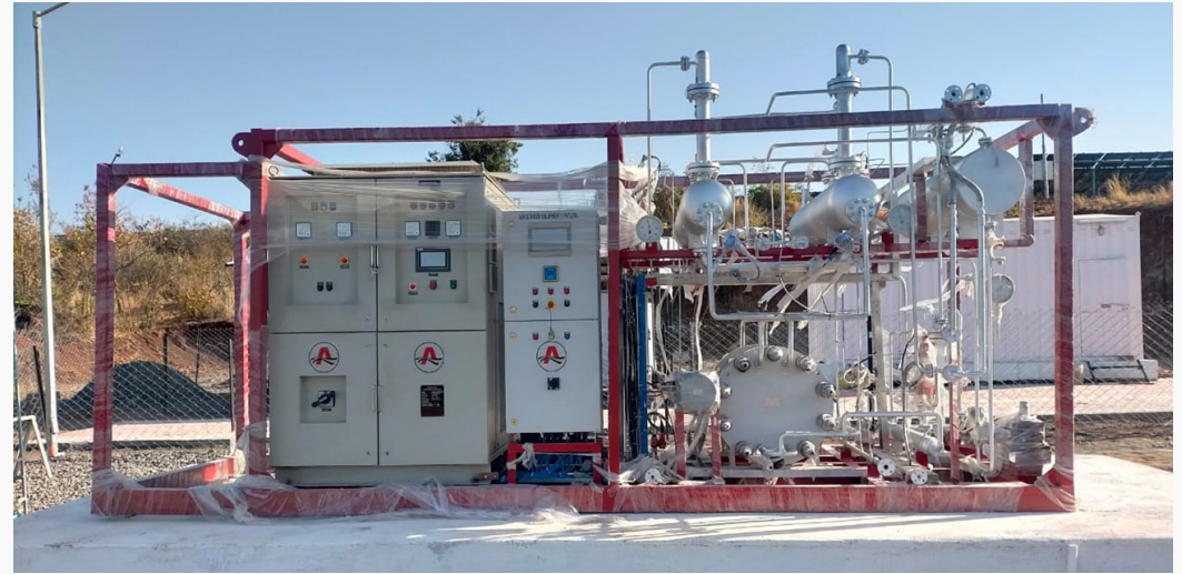
Hygenco - Electrolyser to produce Green Hydrogen under the NEEV Fund
