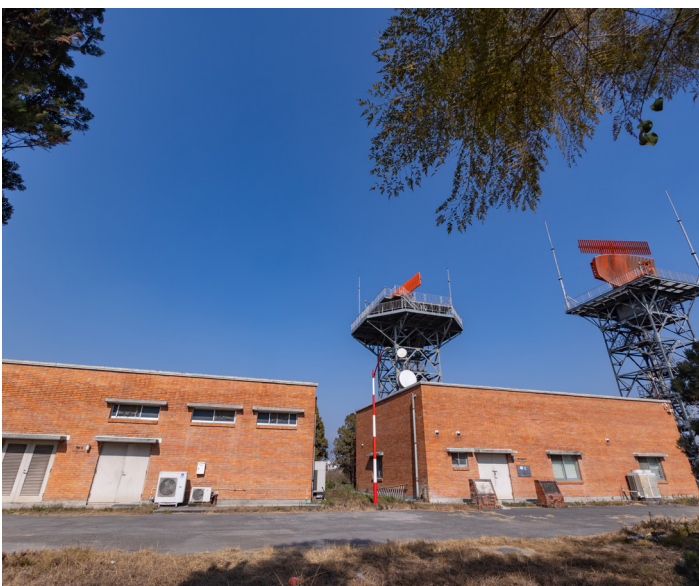
Project for the Modernization of Tribhuvan International Airport in Kathmandu: 1995-97 (Grant Aid Project)
