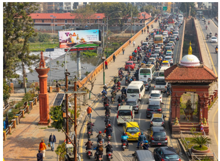
Bagmati Bridge, Kupondol, Kathmandu :1993 (Grant Aid Project)
