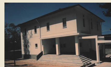
Main approach to Technology Development Building built with Japanese Grant Assistance in Pulchowk, Lalitpur
