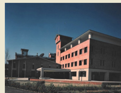
Main building of Water Induced Disaster Prevention Technical Centre built with Japanese Grant Assistance, Pulchowk, Lalitpur
