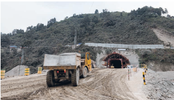
Nagdhunga Tunnel Construction-in-progress
