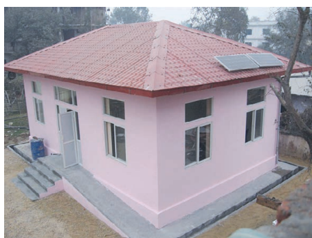
Mediation Center constructed by the SCC project at Dhanusha District Court
