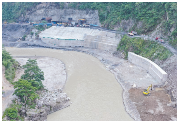
Ongoing Construction work of Tanahu Hydropower Limited
