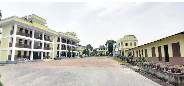
Complete view of ESRP Jyoti Secondary School Building in Harnamadi, Hetauda
