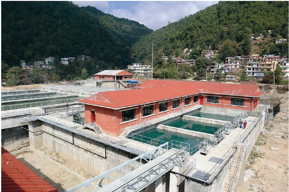
Sundarijal Water Treatment Plant
