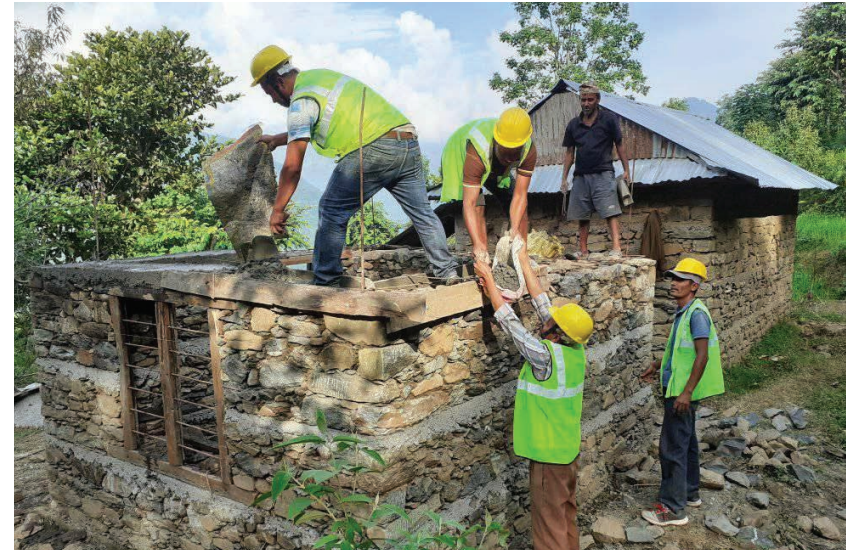
Masons at work in Sindhupalchowk
