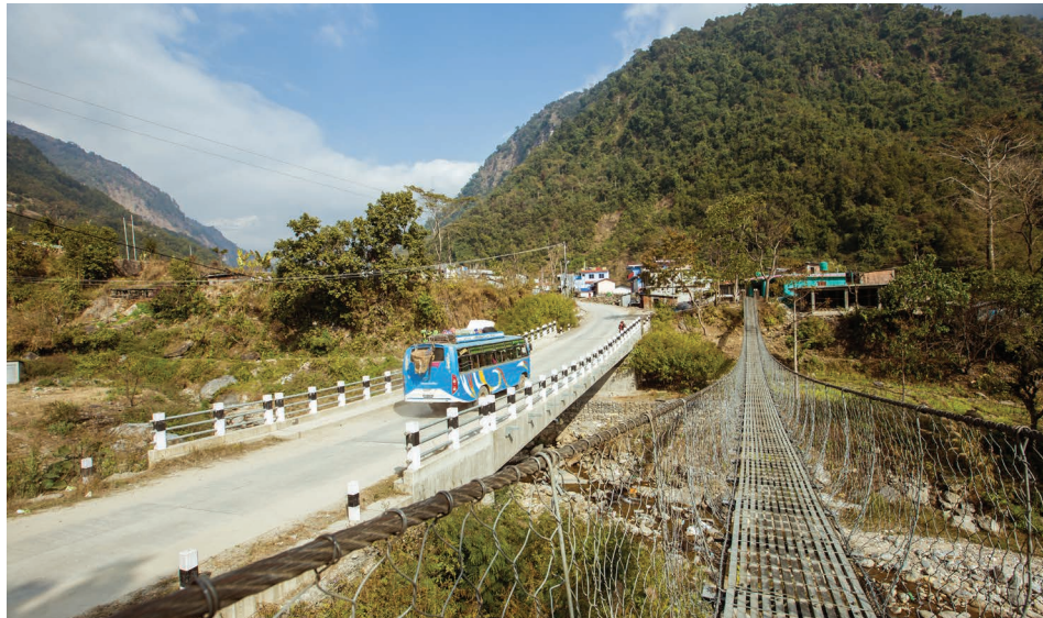
Newly constructed Ghatte Bridge in Gorkha
