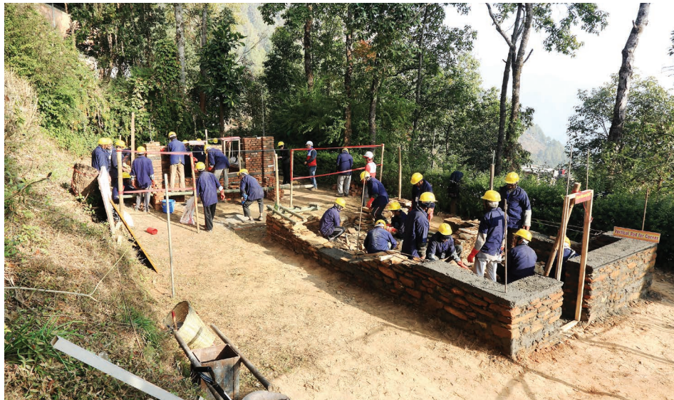
Housing reconstruction training being provided to masons in Sindhupalchowk
