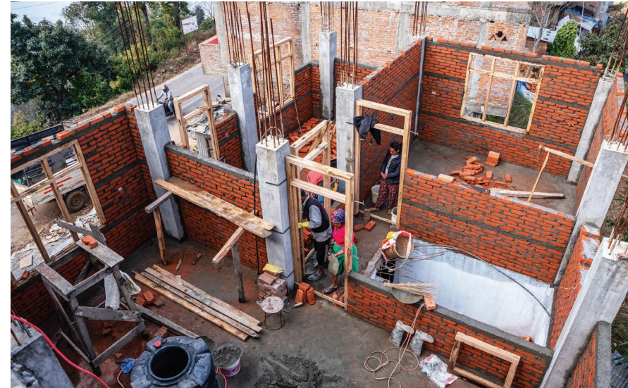
House under construction at Sangachowk, Sindhupalchowk
