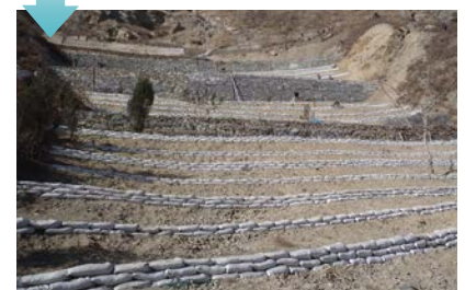
Execution of erosion control work
