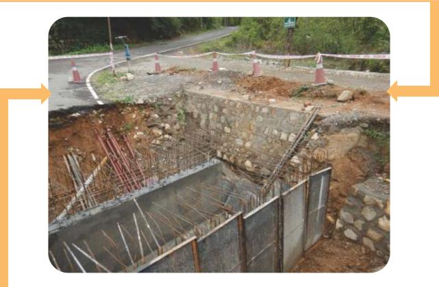
Original road is demolished for the construction of culvert. The road will be restored after the culvert work completes.
