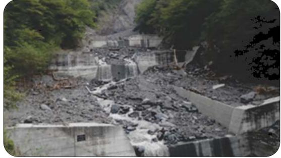
Since the cross section of the dam is trapezoidal, and the valley is an inverted triangle, a dam that extends over a valley requires more concrete as they get higher in height. That is why installing multiple low dams may be more economical than installing a single large/high dam.
