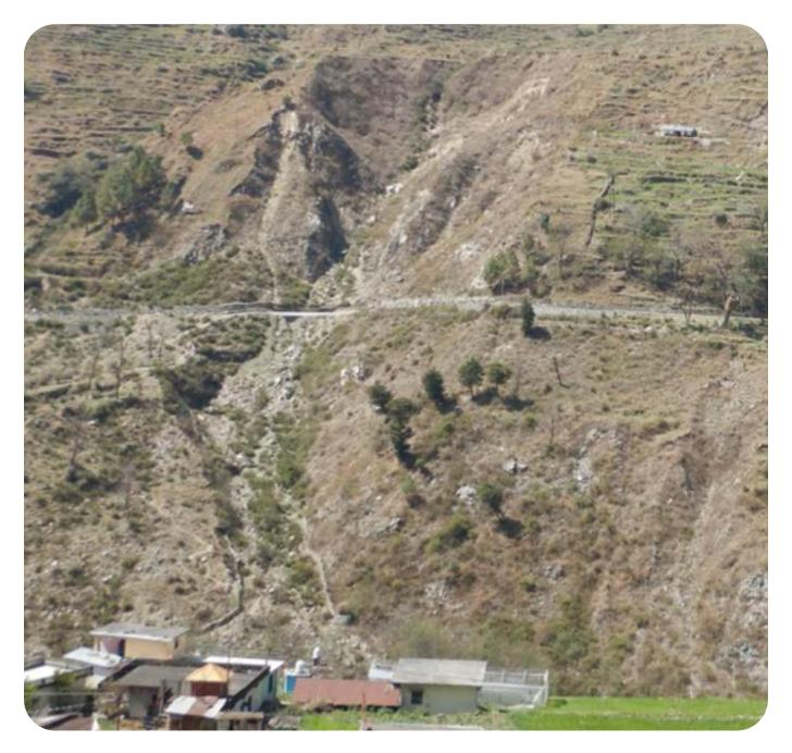
This is a slope failure type disaster site. The site is located at about 26 km from Uttarkashi city on the Uttarkashi – Gangotri Road (National Highway 34). A huge soil mass at the top of the slope had failed and became very vulnerable. Rocks and loose debris had erupted after the slope failure was affected by the subsurface water. The current primary cause of sediment runoff is erosion by surface water during rainfall.
