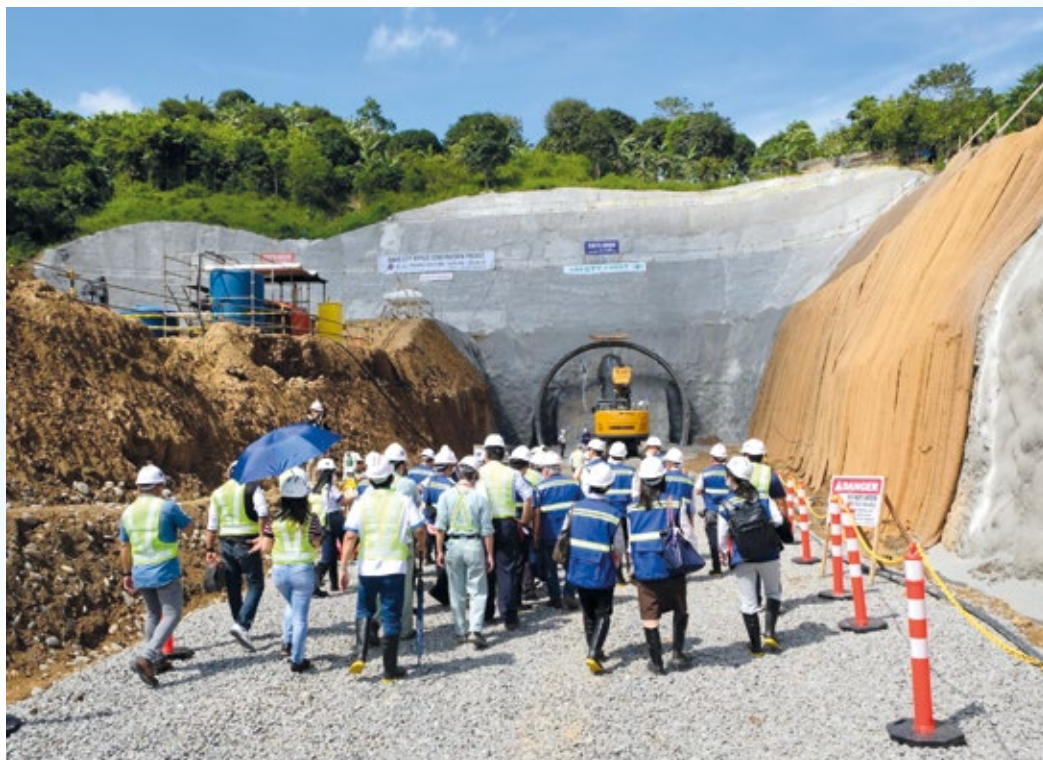
At a joint site inspection of the Davao Bypass
