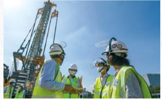
Ongoing construction of the subway
