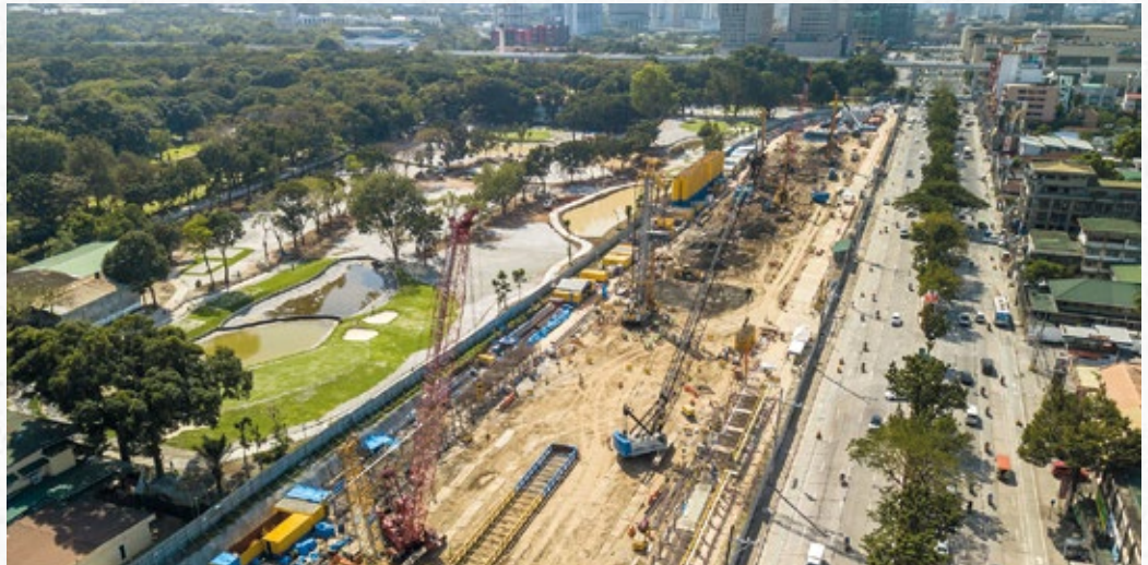
Aerial view of ongoing construction
