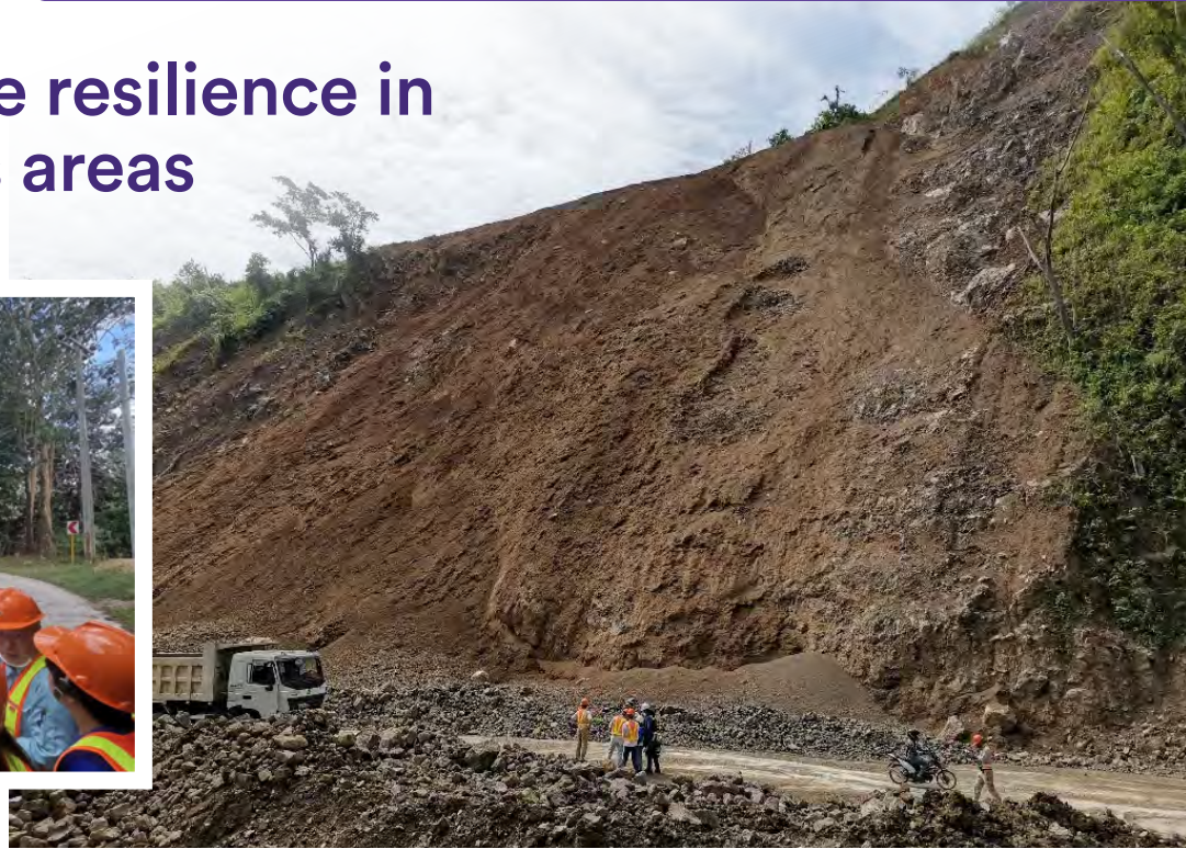
Slope disaster site in Cebu
