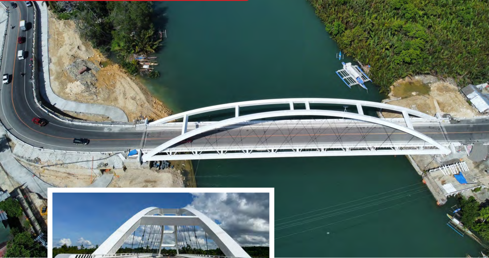
The New Clarin Bridge, Bohol
