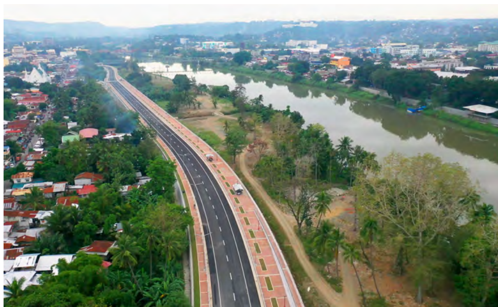
River improvement project along Cagayan de Oro River. Photo courtesy of the DPWH.
