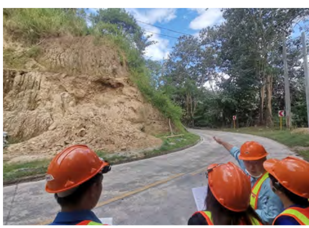
Investigation with DPWH engineers in Baguio
