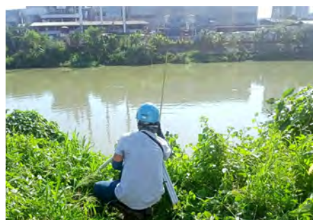
Surveying works. Photos courtesy of the DPWH.
