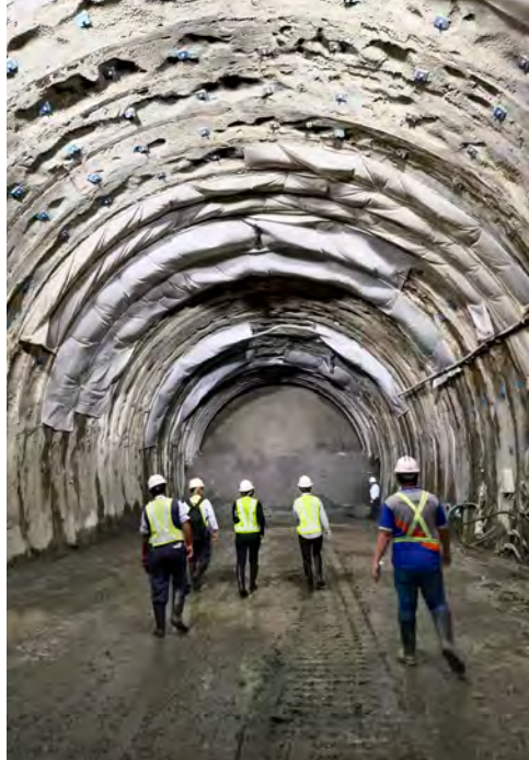
The tunnel can be excavated about 3 meters per day
