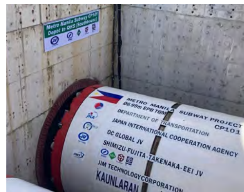
Tunnel Boring Machine
