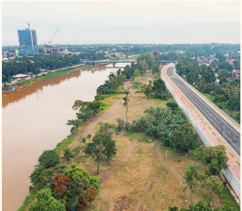
1 Flood dikes and walls built along Cagayan de Oro River.
