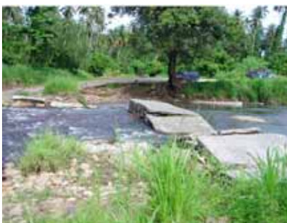
Collapsed Culvert at Rawal
