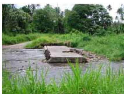
Collapsed Culvert at Warakapis
