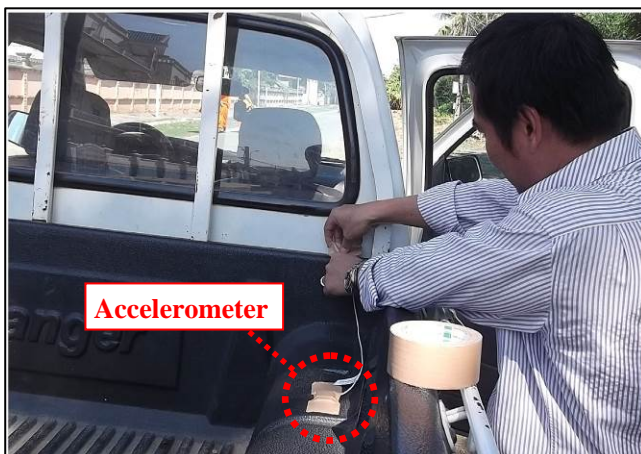
Fig.3 One Scene of DRIMS Installation Work
