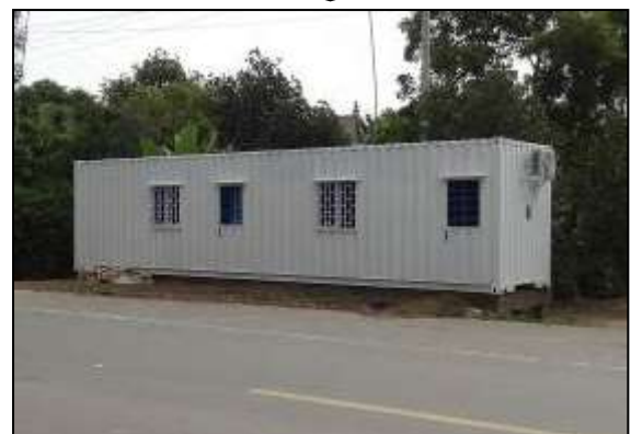
Fig.4 Installation of Container House
