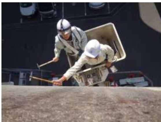
Training by Maintenance Expert
