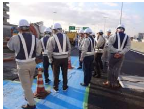
Observation of the maintenance with full stop traffic
