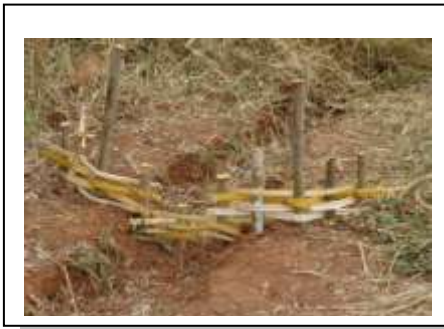
Small Check Dam (Bamboo and poles)
