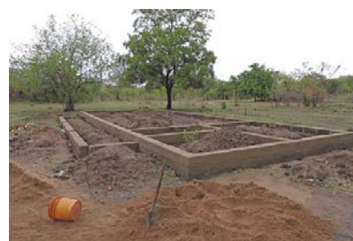
Village office under construction in Tulo village
