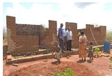
Pre-primary school under construction in Maseyu village
