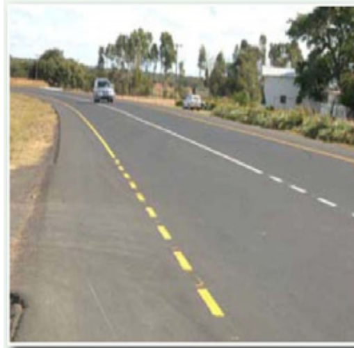
Building of new infrastructure
