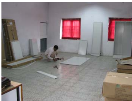
Temporary Office during renovation
