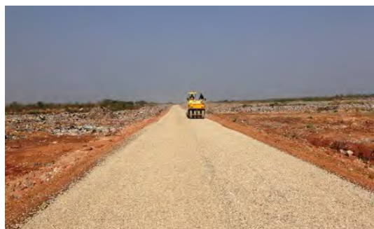
Improvement of access road at KM32 in VTE
