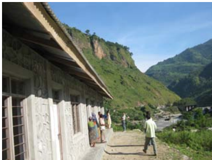
An SOP classroom in the Parbat district. It was built by the community
