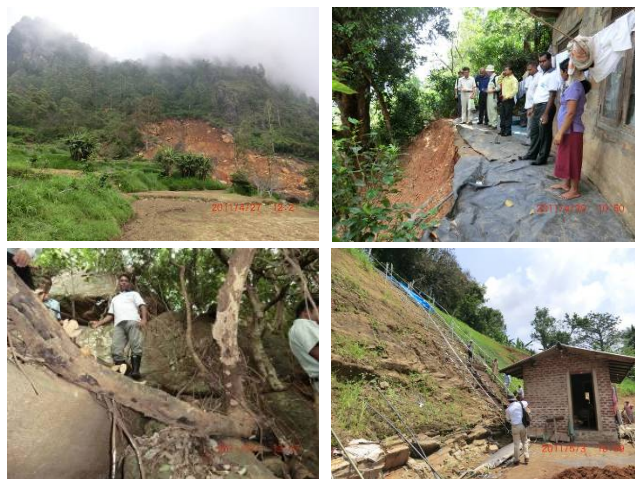
Photos at Central Province
